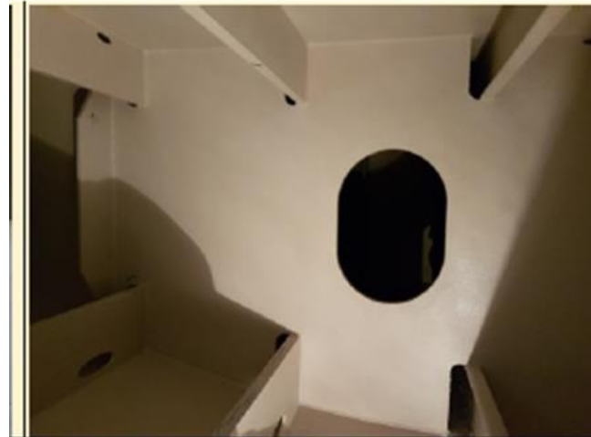
Scrubber Tank 6105, D.F.T. Inspection.
